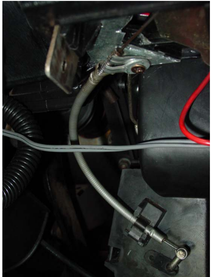
A view from below of the completed, reinforced heater assembly. None of the repairs are visible from the normal cockpit view.
