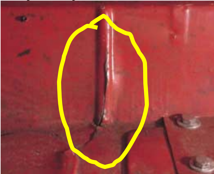
The Crack – post Lime Rock, now a full 8” long!
